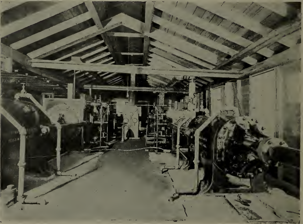
Ingersoll-Rand Corliss Compressor Used in Subway Construction at the Battery Park Plant. This Compressor was one of those used in building the Jerome Park Reservoir.
